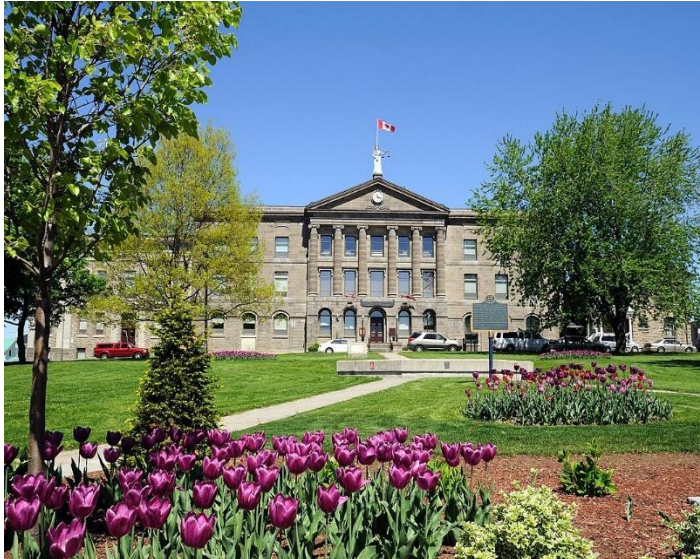
Leeds & Grenville County Court House, Brockville, Ontario
