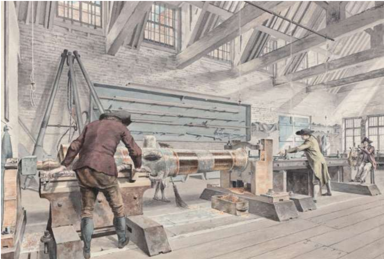
Horizontal boring machine at the Royal Brass Foundry, Woolwich, England c1778 35
