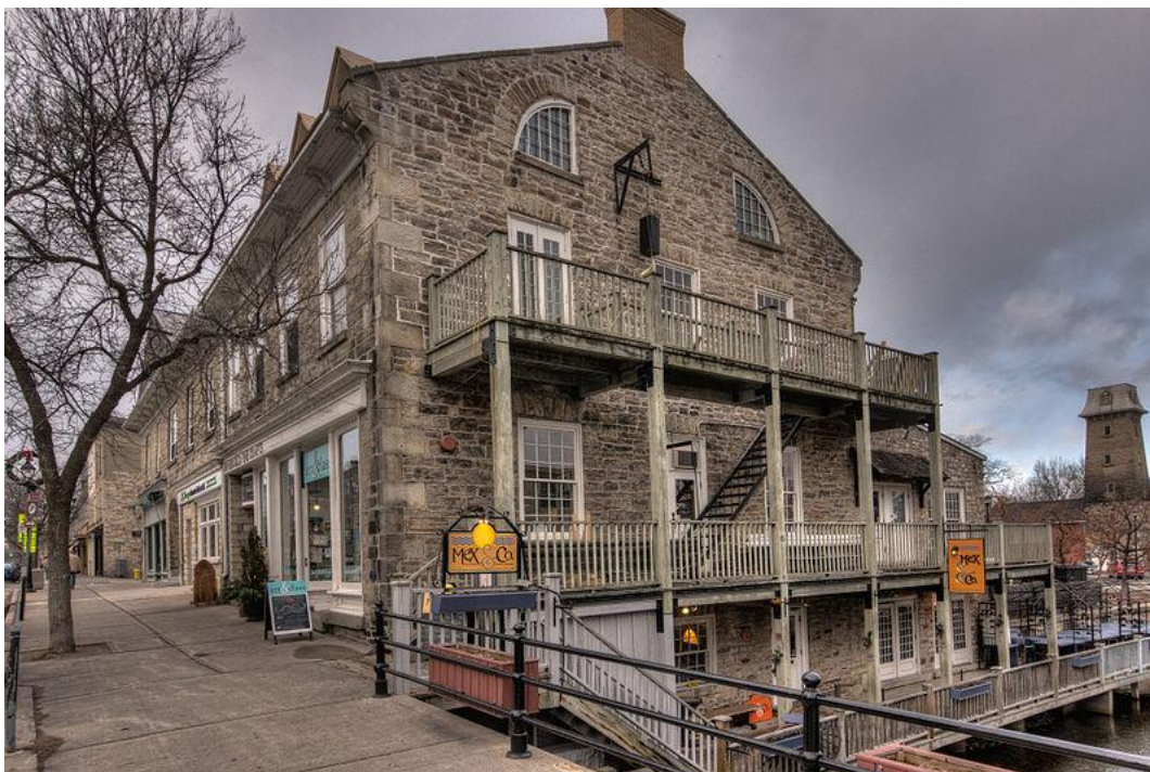
O'Brien Block c2015. In 1860 the Gilbert Barber Shop and sewing rooms were off the lower verandah.
