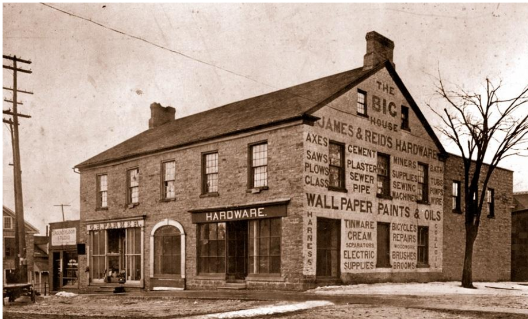
The Graham Block c1901. George Gilbert's Barber Shop was located in the small, single-storey, annex attached to the south (left) end of the building. The Graham building was subsequently replaced by the present building at 44-48 Gore Street East.
