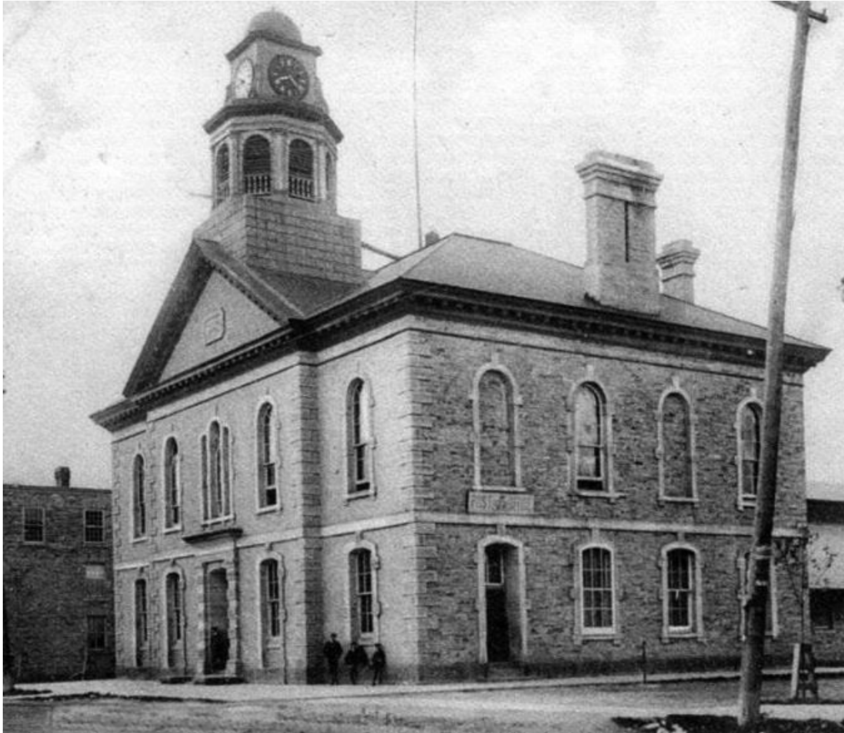
Perth Market Building / Town Hall c1890
