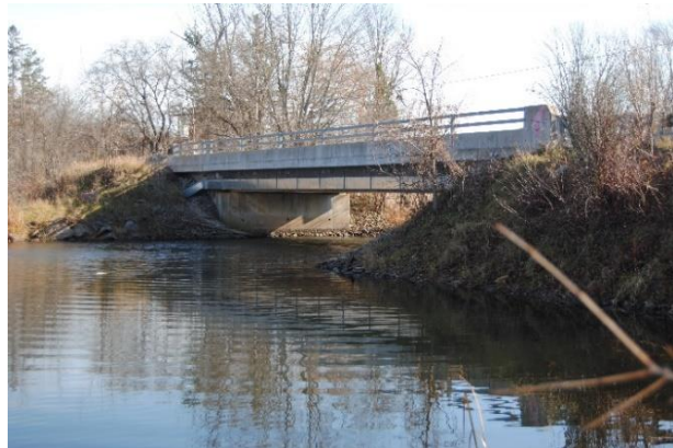
Peter Street Bridge, 2021 (Ron W. Shaw)
