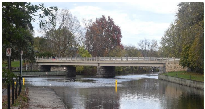
Drummond Street Bridge, Post-1981 (Hamilton Spectator)
