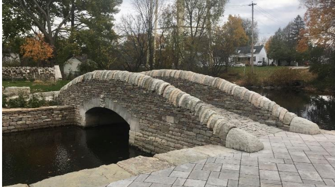
Dry Stone Bridge
