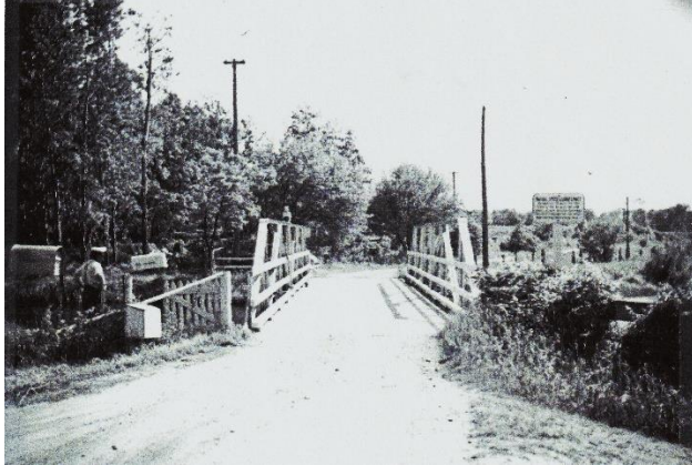
Beveridge Lock Bridge, c1930 (Parks Canada)
