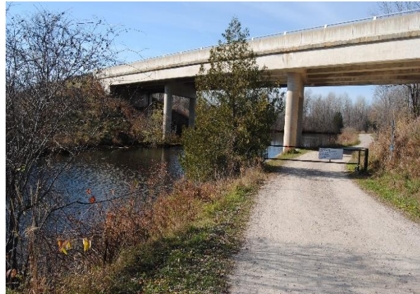
Beveridge Lock Bridge, 2021 (Ron W. Shaw)
