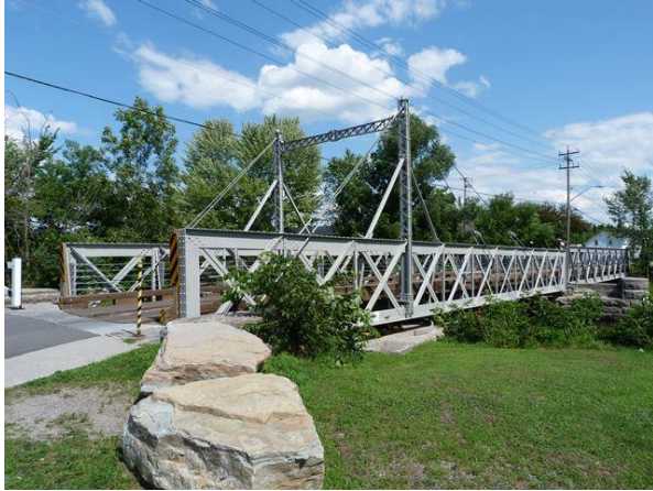
Beckwith Street Bridge, 2013 (Holth & McOmber)
