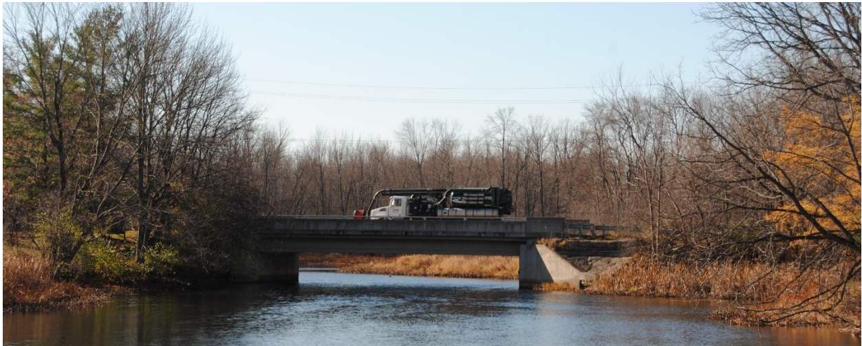
Rogers Road Bridge, 2022 (Ron W. Shaw)
