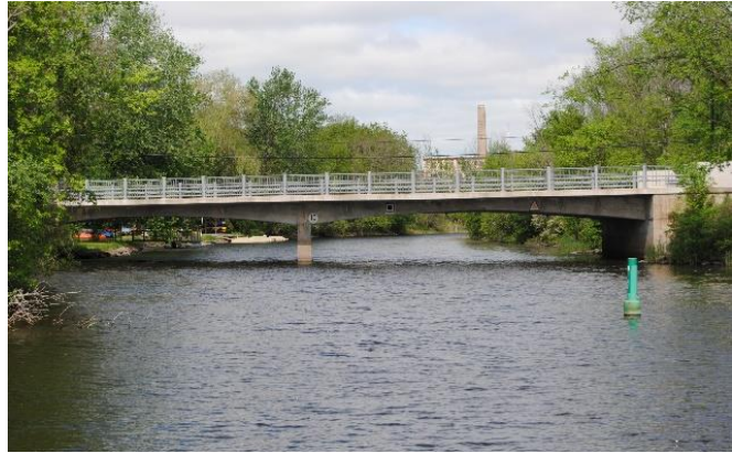
Craig Street Bridge 2021
