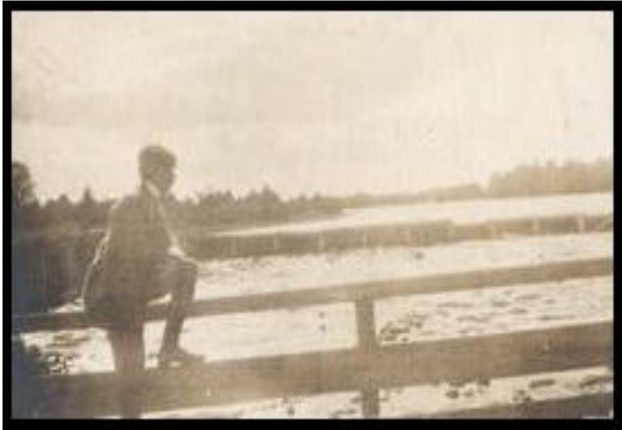
Innisville Bridge and Dam c1907
