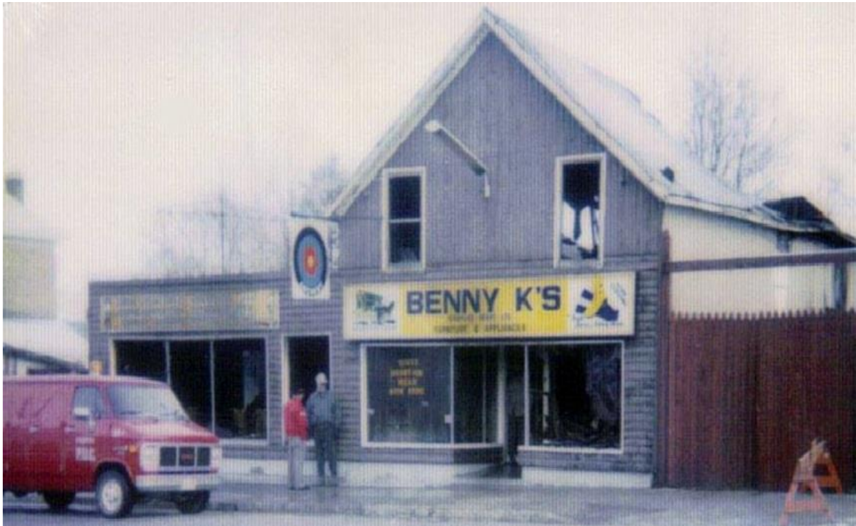
Benny K.'s Gore Street store following the fire of 1991.
