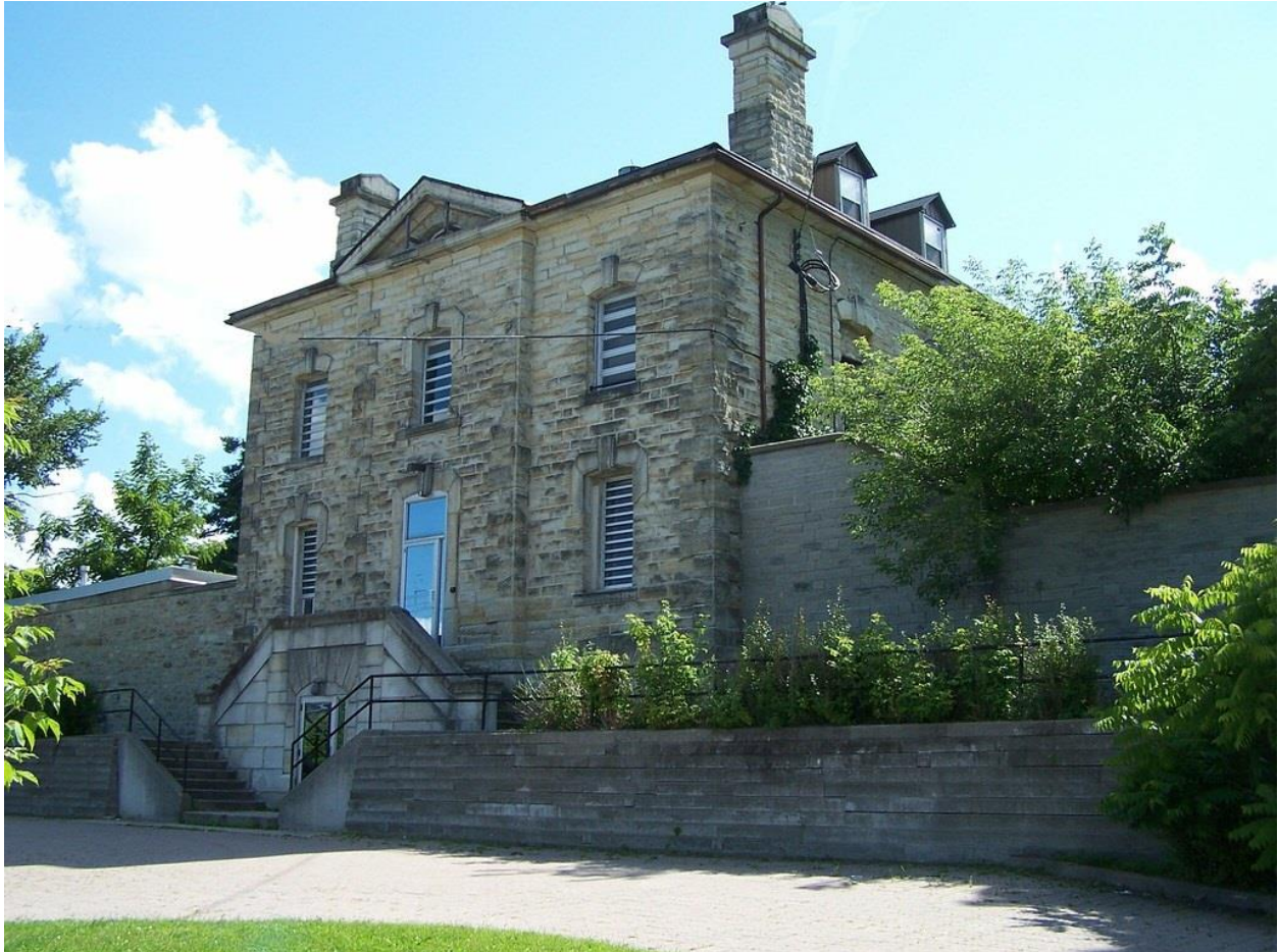
Former Lanark County Jail, Beckwith Street, Perth
