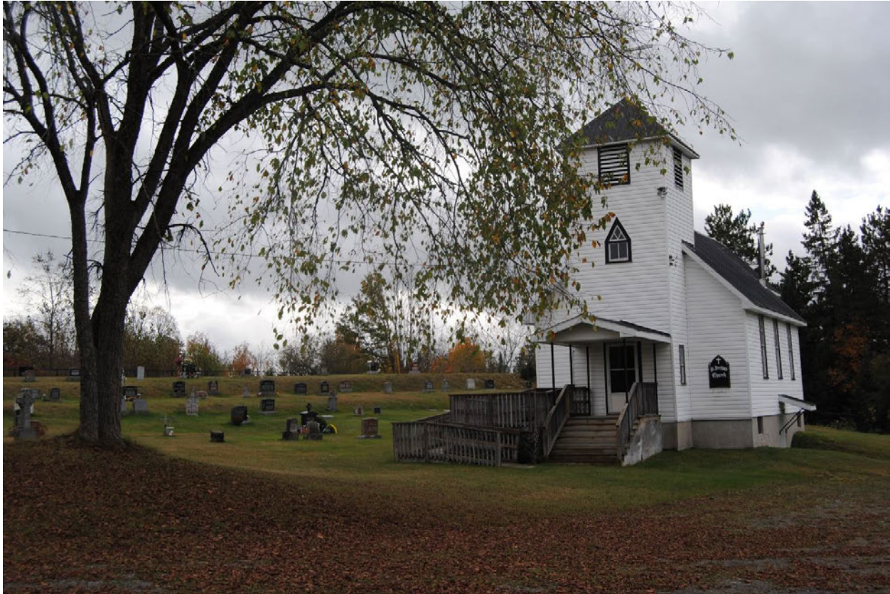
St. Declan's Roman Catholic Church, 791 French Line Road (Photo by the author)
