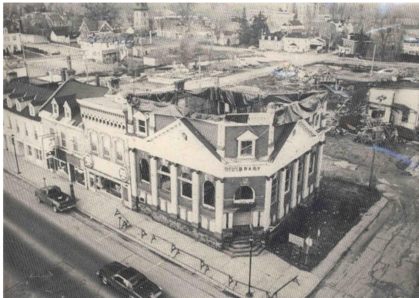
Perth's Carnegie Library after the fire of January 1980. 27
