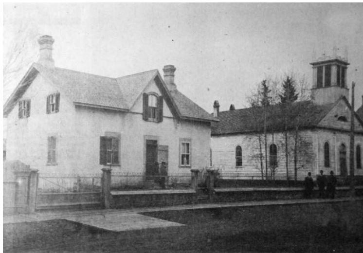
Original Baptist Church and Manse built 1841 (Photo courtesy Perth Remember)
