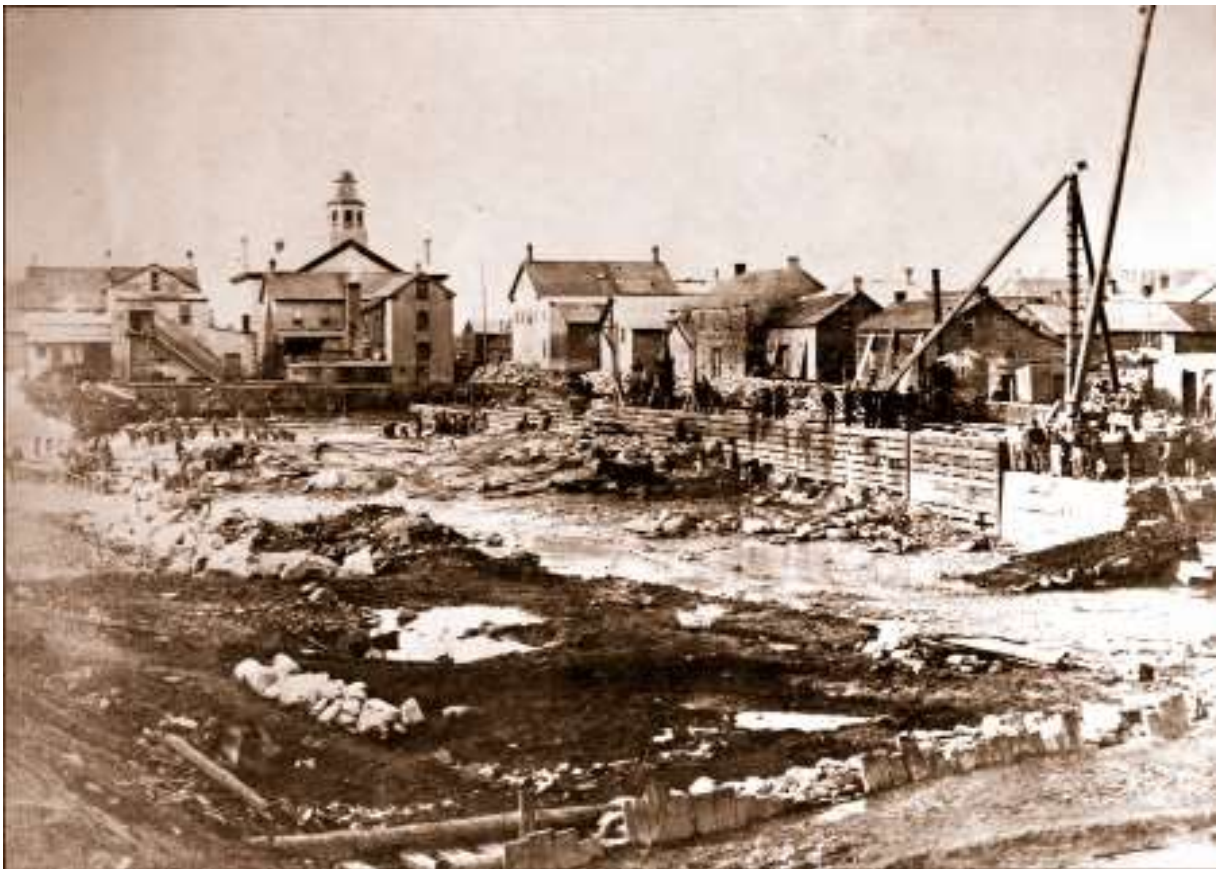
Excavating the Perth Basin, c1891 30
