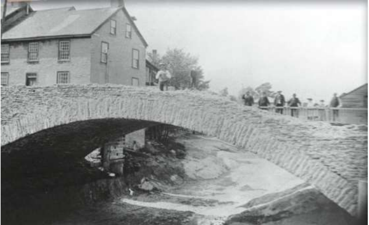
The Gore Street single-arch stone bridge shortly before it collapsed during demolition in 1891. It was being removed to make way for the iron swing bridge on the Tay Canal extension to Haggart's dam. (Photo courtesy of the Perth Matheson House Museum.)
